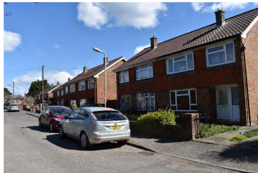
Plate 33: Modern Housing Cellar Hill northern end (facing ENE)
